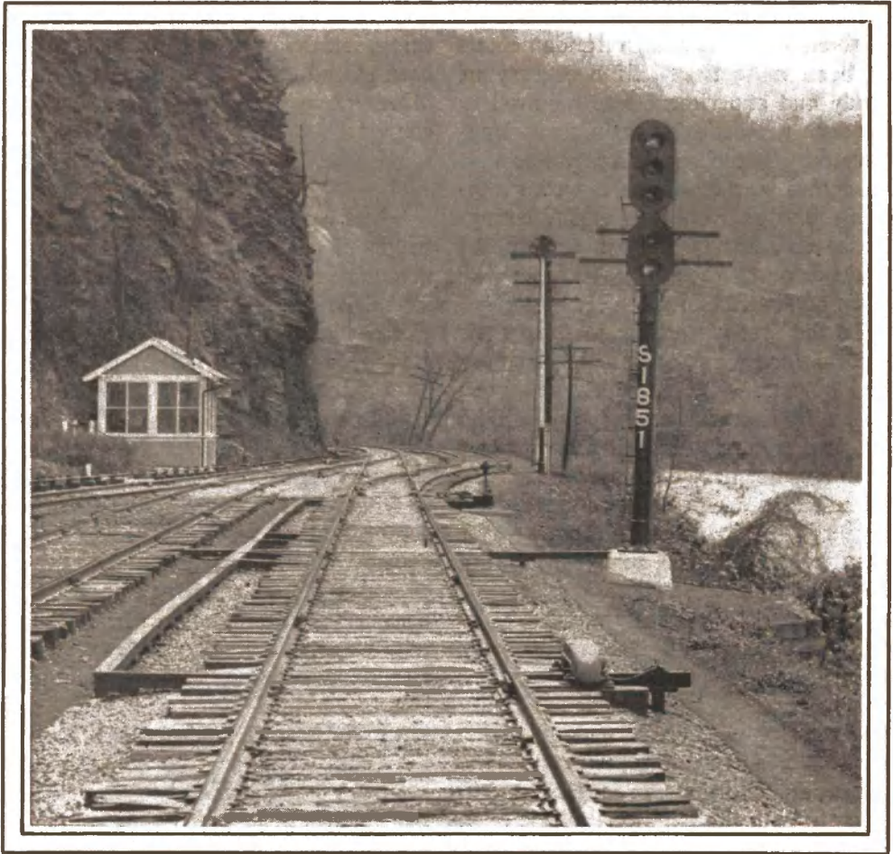
Photo by Courtesy General Railway Signal Company.
